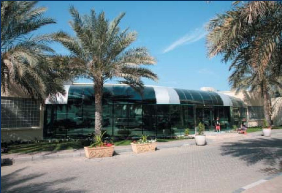
Gymnasium Refurbishment at Le Meridien Mena Seyahi
